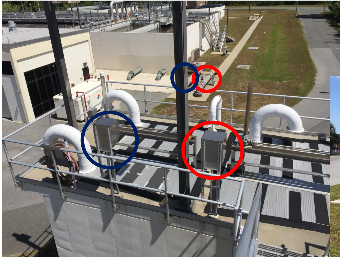
Anastasia Island 20" Ductile Iron Pipe Cement lined Raw Sewage
